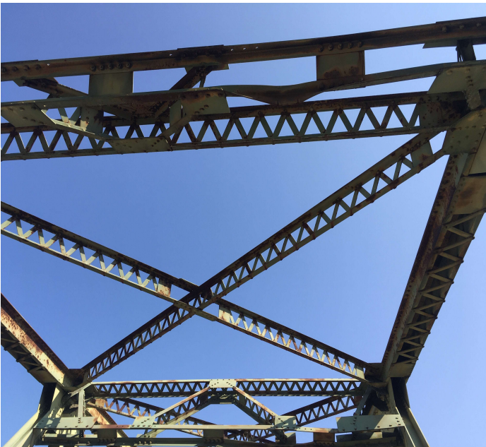
PHOTO 3 Description Portal brace damage at beginning of the truss. U8
