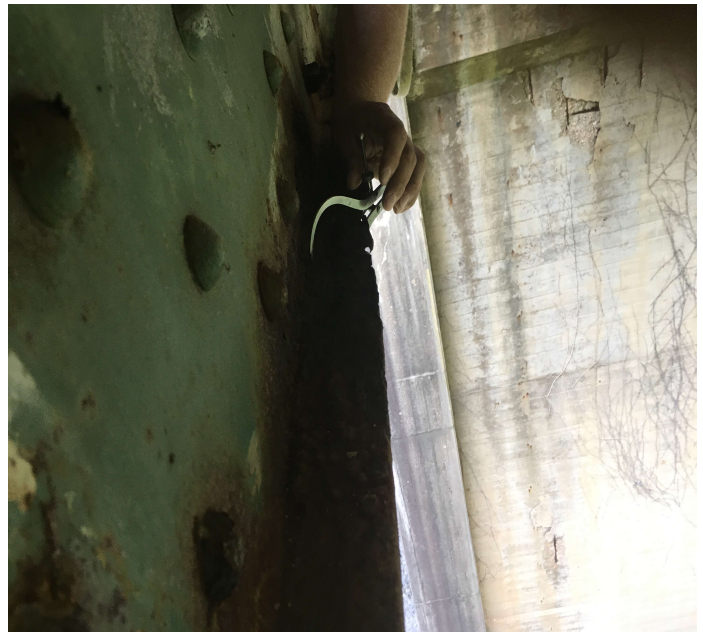
PHOTO 2 Description Section loss on the interior bottom chord flange at L 26. The remaining section is 5/8" next to the web down to knife edge at the edge of the c-channel flange for a length of 8";
