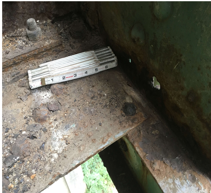
PHOTO 1 Description 1" and 1/4" rust holes in the vertical gusset plate at the back side of L6 right truss at the bottom chord. The gusset plate has 1/4" section loss for 13" on the interior side. The original gusset plate thickness is 3/8" thick.
