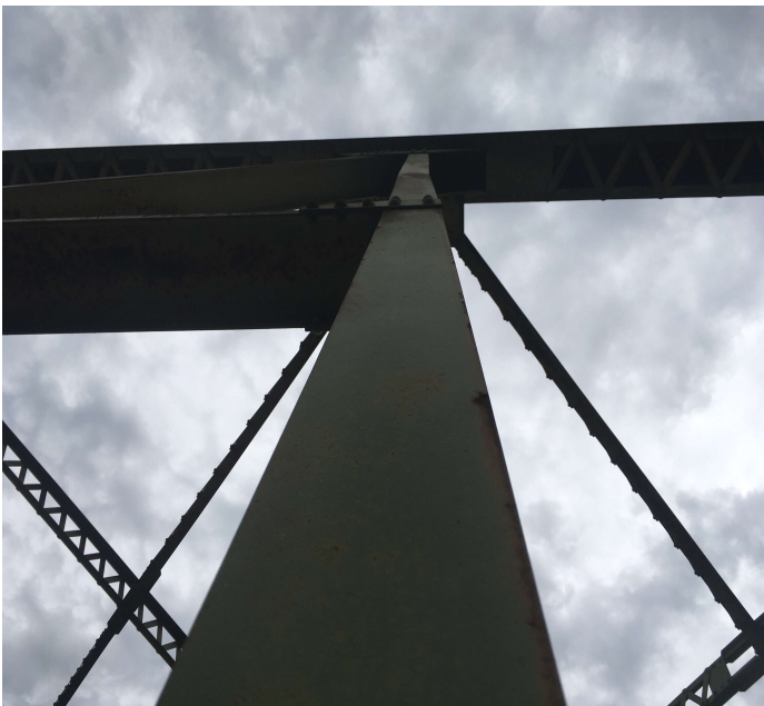
PHOTO 1 Description Out of plane bending at the U12 vertical due to the lateral bracing having vehicle impact damage.
